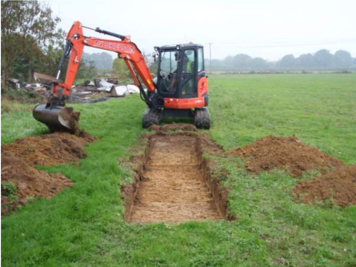
Plate 1 – Trench 1 under excavation (looking ENE)
